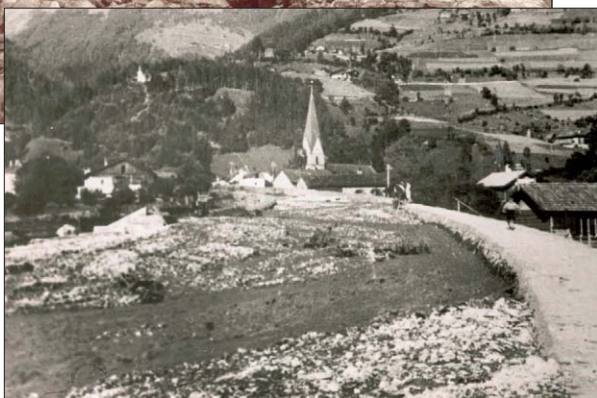
Abb 3: Since 1884 torrent control measures were done.
