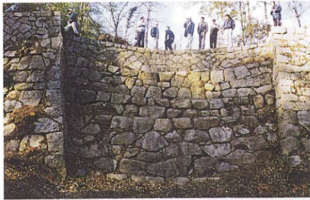
Photo-1 Fukami sand retaining works – This dam was constructed by stone masonry in Dodo River in 1854 (Hisoshima Prefecture)
