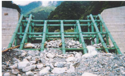
Fig.1 Open type steel check dam
