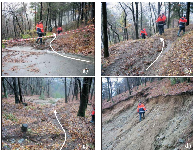
Fig4: Frana di Ponte Valtellina: il ruscellamento delle acque non incanalate come causa scatenante (vedi testo) Fig4: Ponte Valtellina landslide: in corrispondenza di a sharp turn of the road part of the water flowing on the concrete paving (a) is diverted, because of the presence of an obstruction in the culvert, along a dirt pathway (b) and finally in the slope below (c). This water gave a crucial contribution in the saturation of the soil cover, inducing the slope collapse (d).
