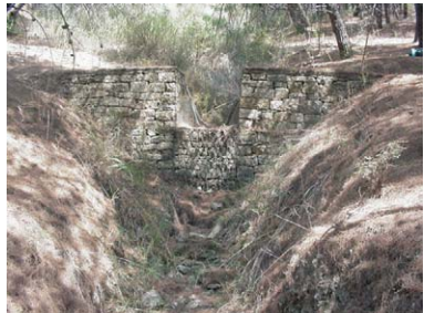
Fig. 5 - Briglia in gabbioni Fig. 5 - Gabion check dam
