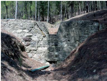
Fig. 4 - Briglia in pietra e malta Fig. 4 - Stone masonry check dam
