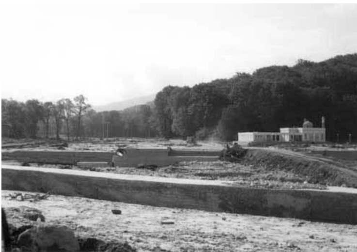
Picture 1 Human encroachment to main river frontage
