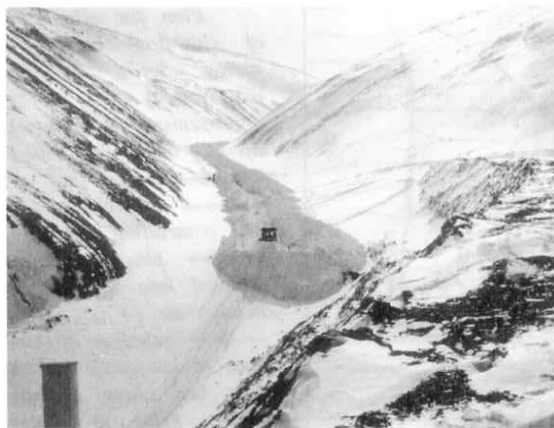
Fig. 4 Permanent slushflow hazard mitigation. Removal of snow from the potential starting zone and track in Vannledningselva, Longyearbyen, Svalbard, is done every spring to protect the development area on the fan. The rockfill in the right half of the picture is part of a huge direction control work. (Photo E. Hestnes, NGI)
