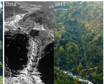
Dorodani Sabo Dam Group Revitalizing the Greens
