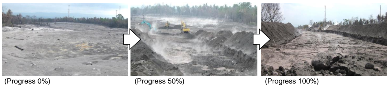
Fig. 6 Situation of the construction work
