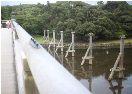
Fig. 1 Traditional Japanese technique to prevent damage to historical bridges using stakes, Upper: Togetsu Bridge, Arashi-yama, Kyoto; lower: Uji Bridge, at the Ise shrine, Mie
