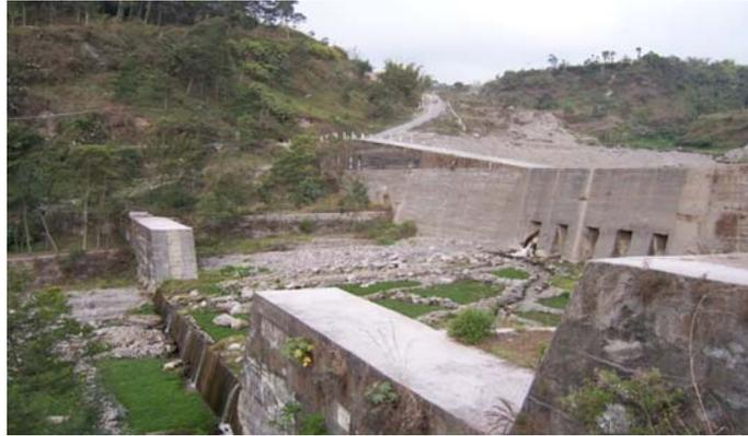
**Fig. 5** One of the check dams in Mt. Merapi area has another function as a submerged bridge (Photograph taken by Agus Sumaryono)
