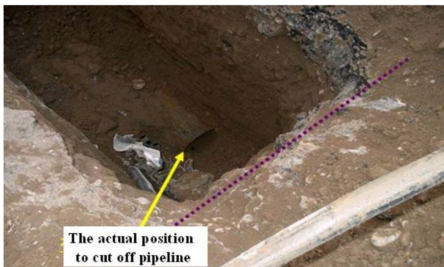
Figure 10. Photo of excavation result
