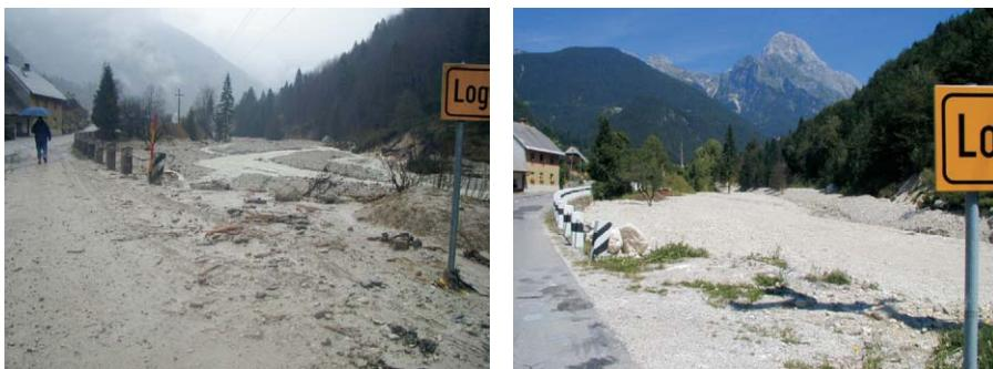
**Fig. 5:** A view towards the Koritnica River channel in Log pod Mangartom immediately after the debris flow event in November 2000 and after the completion of the first river engineering works in July 2001.
