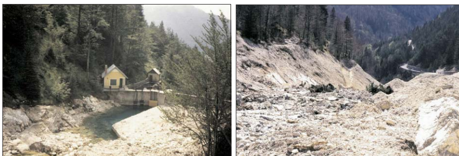
Fig. 3., 4: The hydropower plant object in the torrent Mangartski potok before and after the debris flow (Photo: archives of the PGD Log pod Mangartom)
