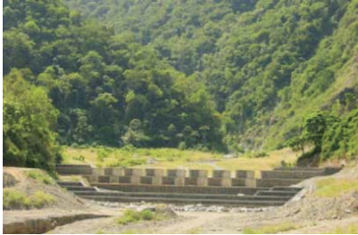
Fig2: Open dam in Piedra Azul torrent. (2003)
