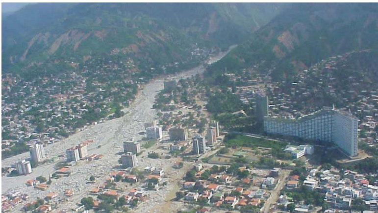
Fig1: Debris cone in San Julian torrent, January 2000 (Source: UCV)
