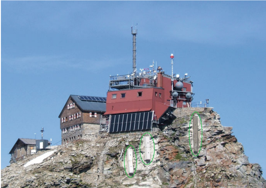
Fig. 4 Completes adaptation works at Hoher Sonnblick observatory (3,106 m a.s.l.) to reduce problems of permafrost degradation (picture by Schöner W.)
